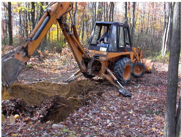
Photo 9 – Test Pit Excavation
